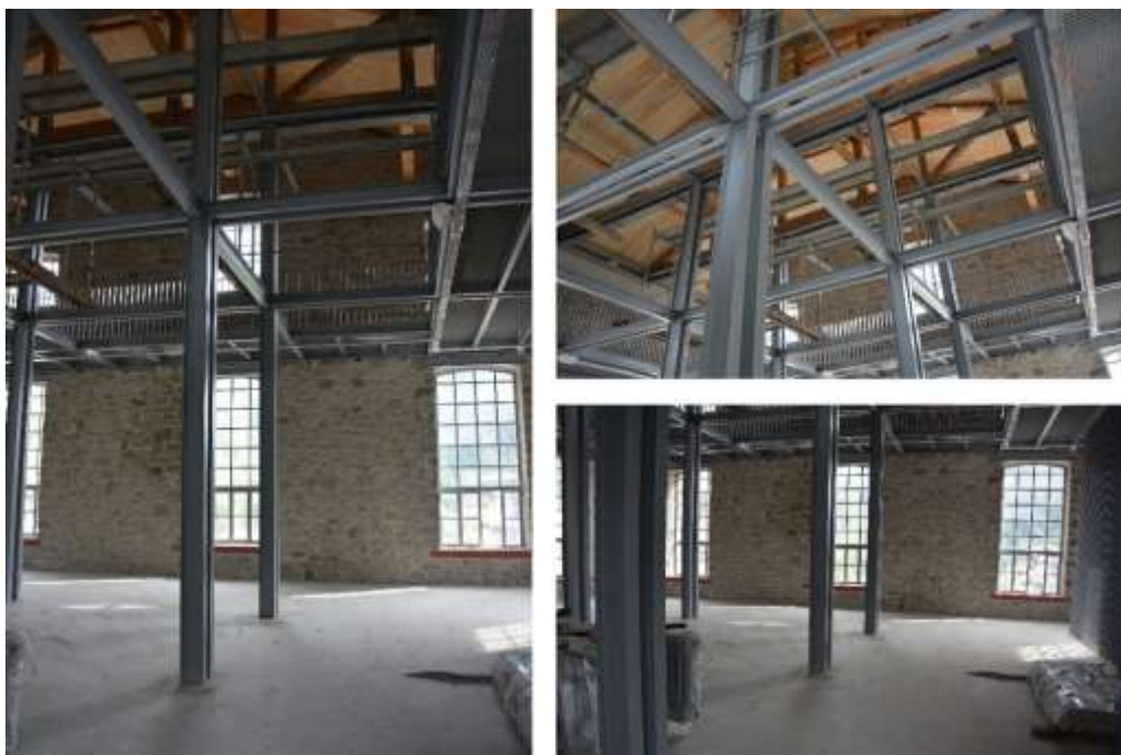
Photo 8: Lavuar Building -View from the Upper Ground Level.
