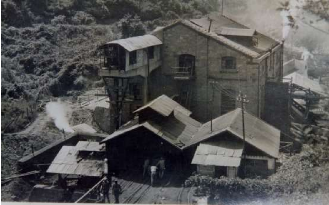
Photo 2: Asma-Dilaver Hard Coal Operation Management Coal Washing Building. Source: TTK Archives.
