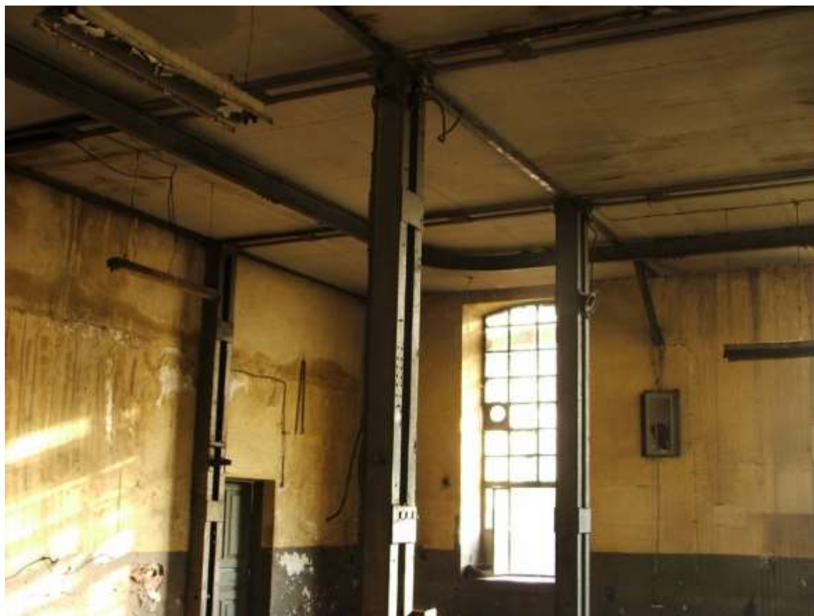
Photo 4: Interior of the Asma-Dilaver Hard Coal Directorate Washery Building. Sourc: Muhsin Maden Archive, 13.02.2004.
