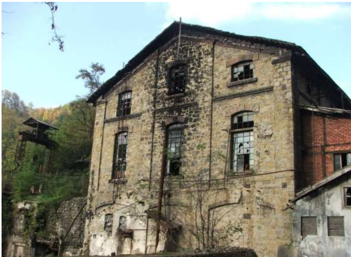
Photo 3: Asma-Dilaver Hard Coal Directorate Washery Building. Source: Muhsin Maden Archive, 13.02.2004.
