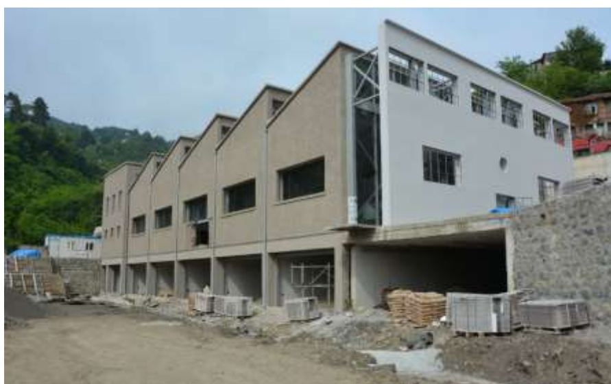
Photo 9: Workshop Building -View from the Upper Ground Level.
