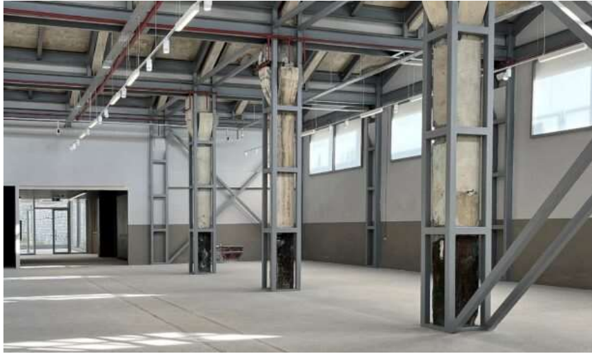
Photo 10: Workshop Building -Multi-purpose Hall on the Upper Ground Level.
