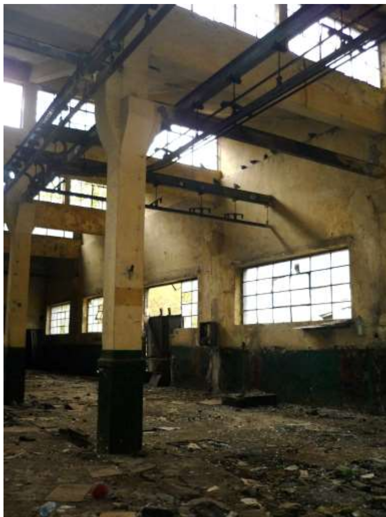
Photo 6: Interior of the Asma-Dilaver Hard Coal Directorate Workshop Building. Source: Muhsin Maden Archive, 13.11.2008.
